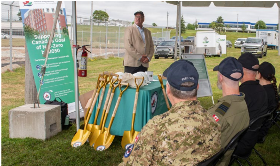
Project Manager Peter Doggett speaks at the groundbreaking event for the new solar array field being built near the entrance of 12 Wing Shearwater.
