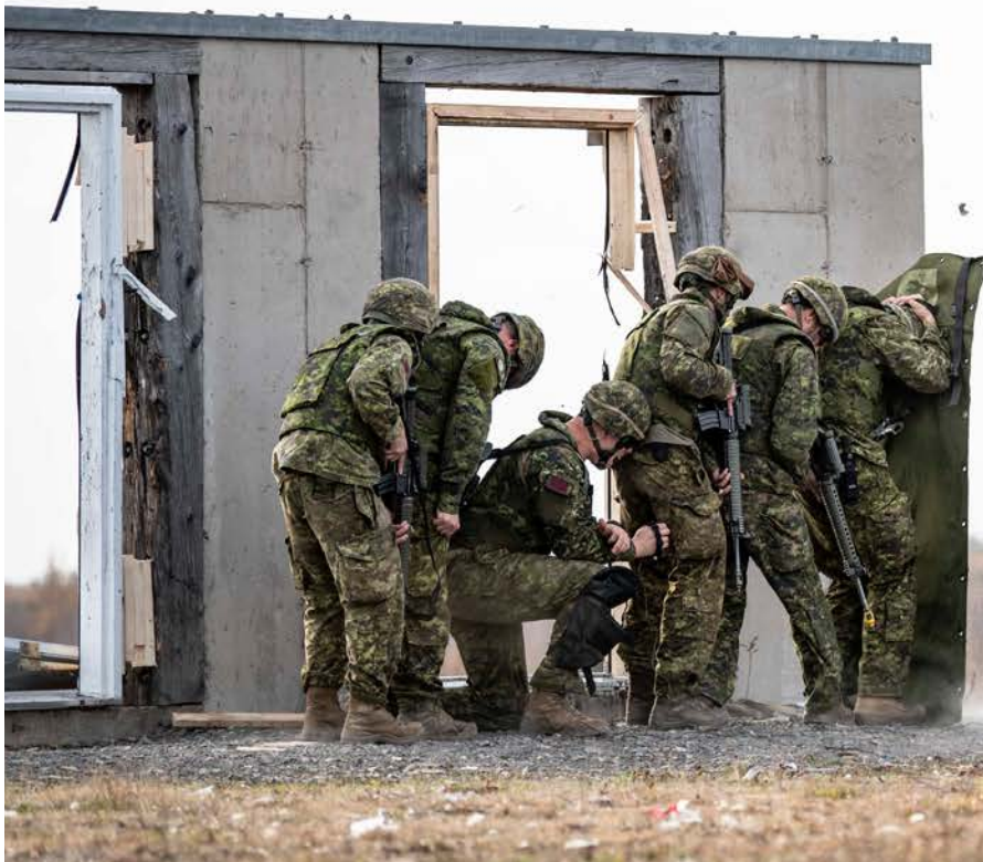
Members of 4 Engineer Support Regiment (4 ESR) perform explosive breaching during Exercise Nihilo Sapper at 5th Canadian Division Support Base - Gagetown on November 6.
