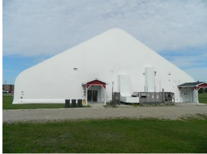
CFB Borden Fitness Facility
