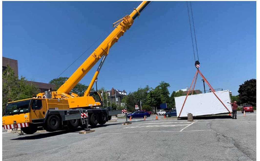
A crane places a CT scanner into the parking lot of CF H Svcs C (A) at Stadacona on June 19, 2020.
