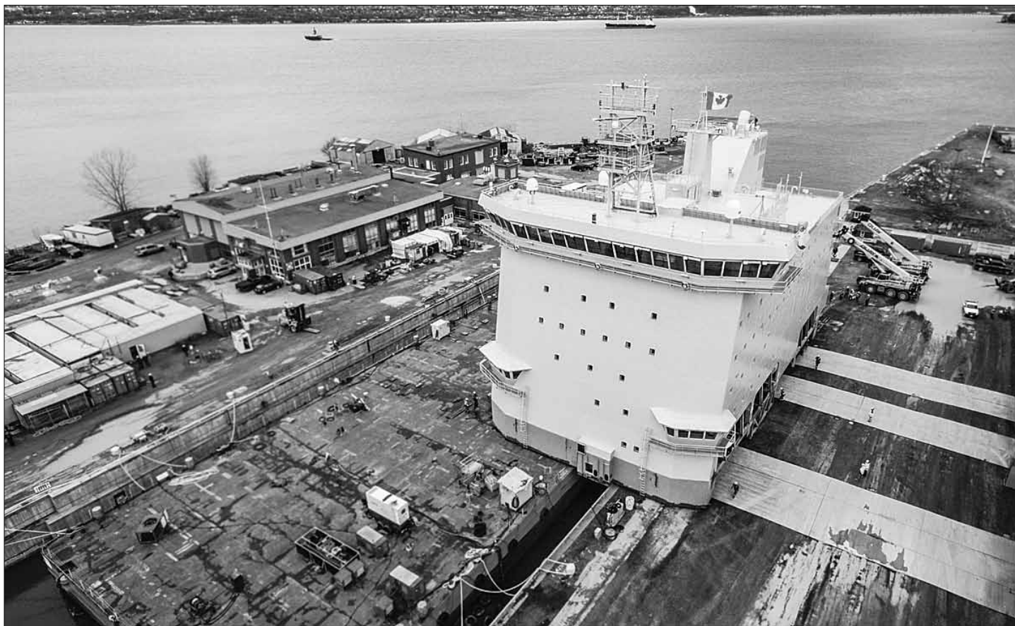
The newly-built accommodation superstructure was recently lifted and transported onto the MV Asterix, which is being converted by Davie Shipbuilding in Quebec to deliver interim AOR capabilities to the RCN. The vessel is expected to be delivered to Halifax in September.
