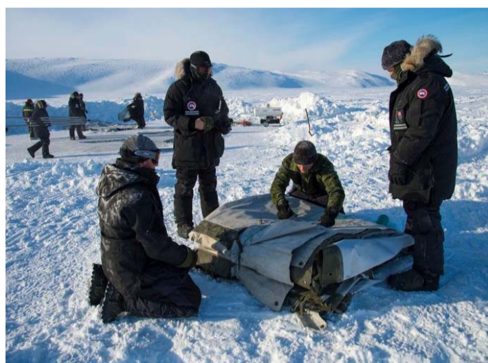
Clearance Divers and Port Inspection Divers from FDU(A) take down the dive site after completing the fresh water pipe inspections at Canadian Forces Station ALERT during Operation NUNALIVUT, April 9, 2016.
